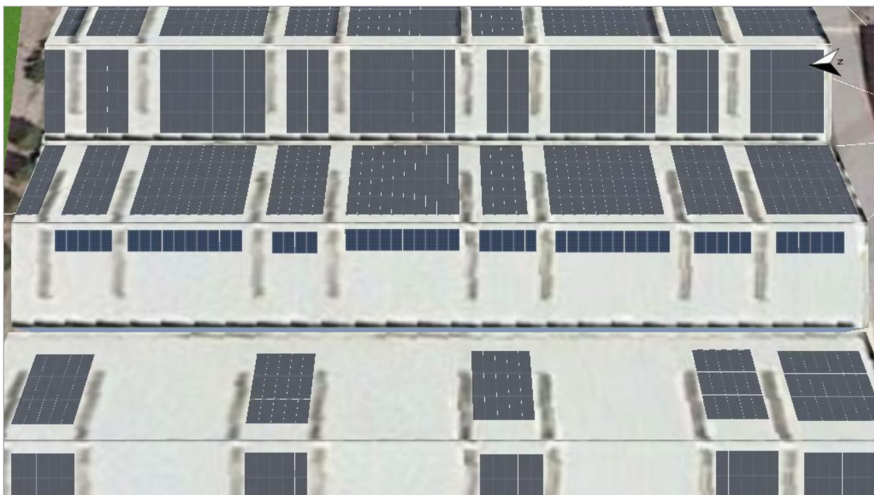
Figure: 7. Module Area - Building 03-Roof Area West
