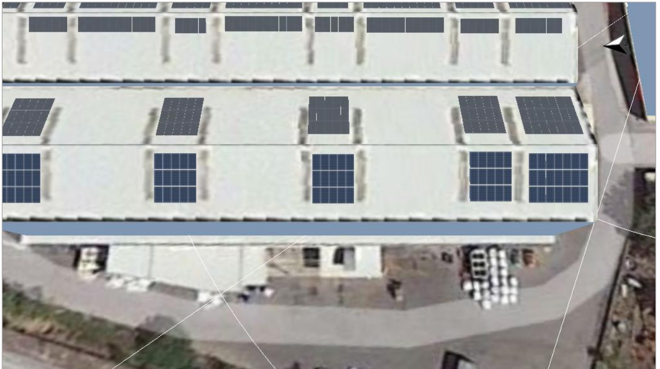
Figure: 5. Module Area - Building 05-Roof Area West
