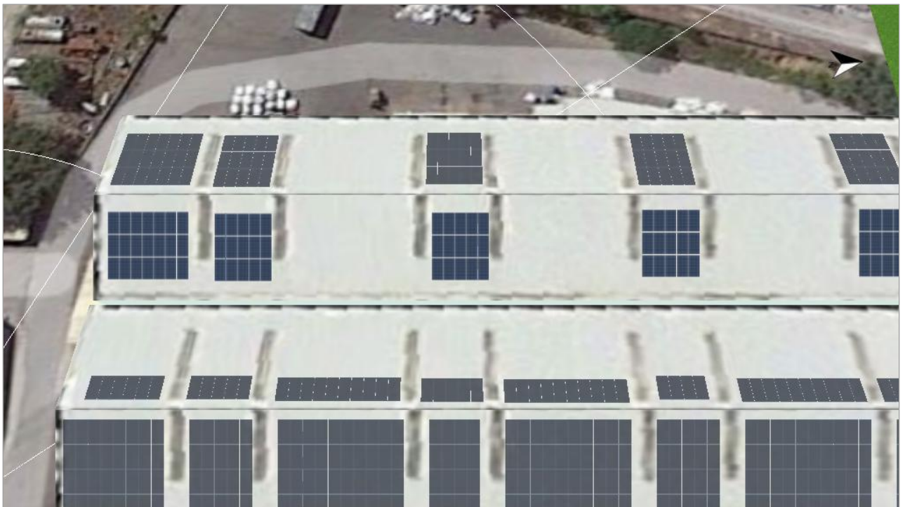
Figure: 6. Module Area - Building 05-Roof Area East
