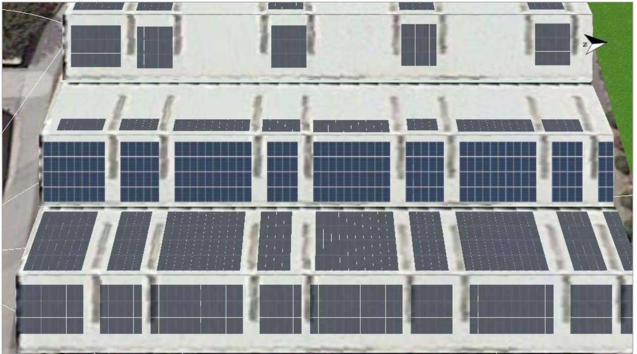
Figure: 4. Module Area - Building 03-Roof Area East
